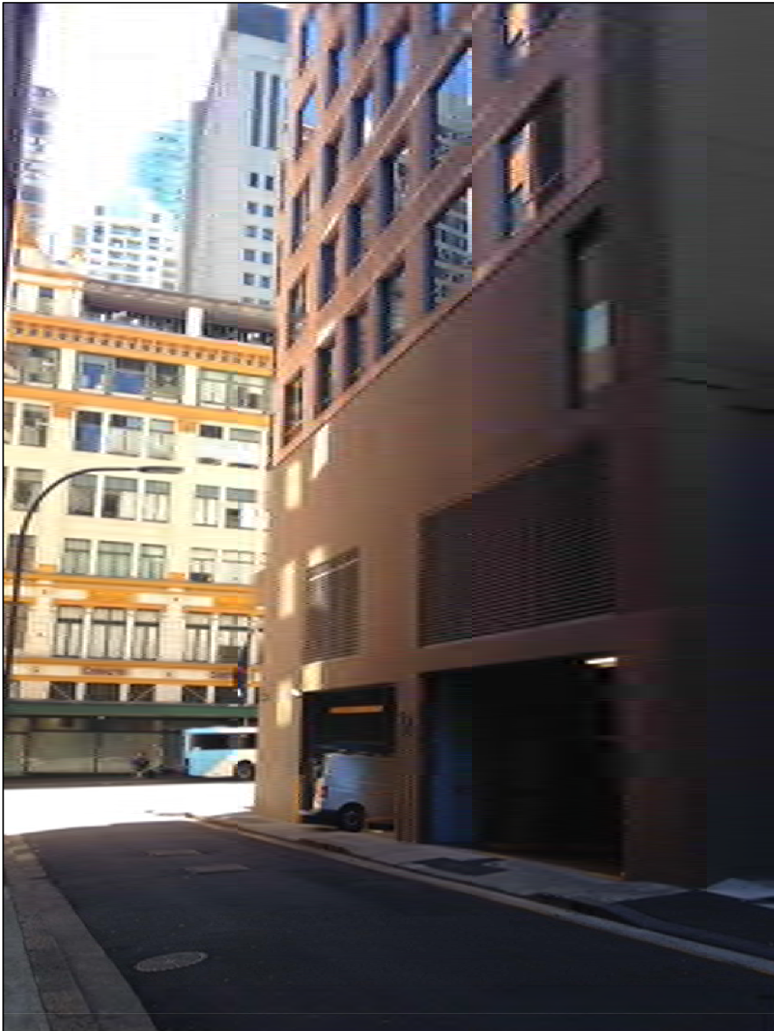
Figure 4: The existing vehicular access to the site from Clarke Street
